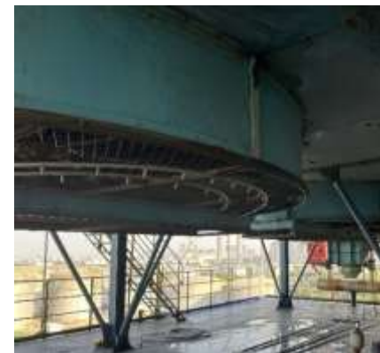
重整工艺空冷器间接喷雾降温 Indirect spray cooling for the air cooler in reformer unit
